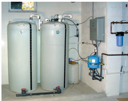
Figure 2. Well system with atmospheric storage
