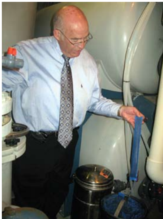
Dr. David Knighton, who 'discovered' the water treatment and conditioning properties of sphagnum moss, examines a moss refill that helps control biofilm formation in the children's activity pool at the Highland Park Aquatic Center. (Photo credit: Laurel Edwards, City of Saint Paul Parks and Recreation)
